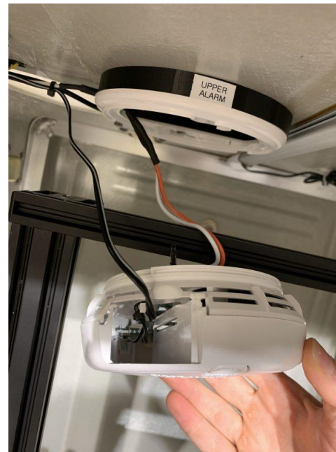
Hard-wired smoke alarm with printed mount bracket
