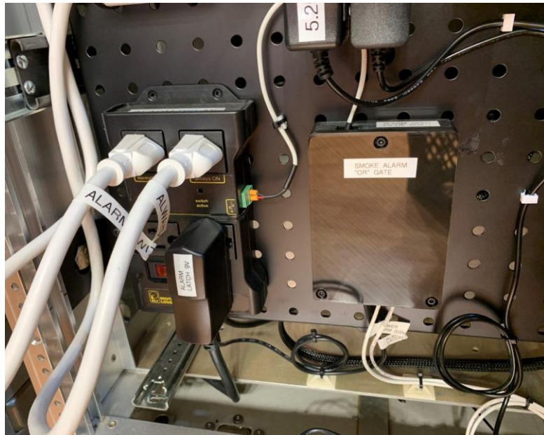
PCB enclosure with power relay
